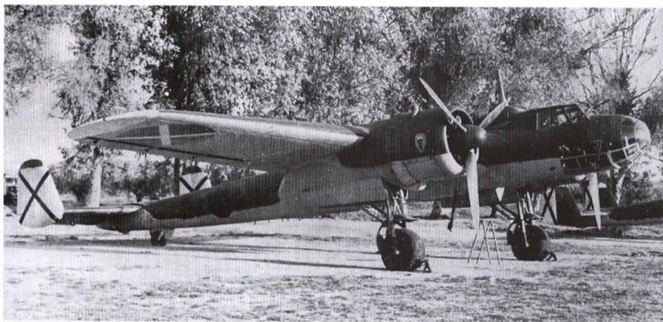
43 Above: A view of 27-29 which shows the Bramo radial engines of the Dornier Do 17P to advantage. These later models also received the devils head emblem on their cowlings
