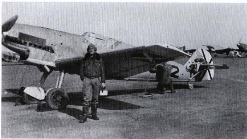
131: An unidentified pilot poses in front of a Bf 109D, 6-52 of 2.J/88. The aircraft is probably finished in RLM 02 and 65 and has a single white victory bar on the fin. Note that it is not fitted with a radio mast
