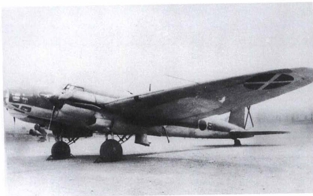
332: This is Heinkel He 111E, coded 25-81, showing the drag-producing ventral bath tub. The 2.K/88 badge is visible on the nose. The unit was also distinguished by its red propeller spinners
