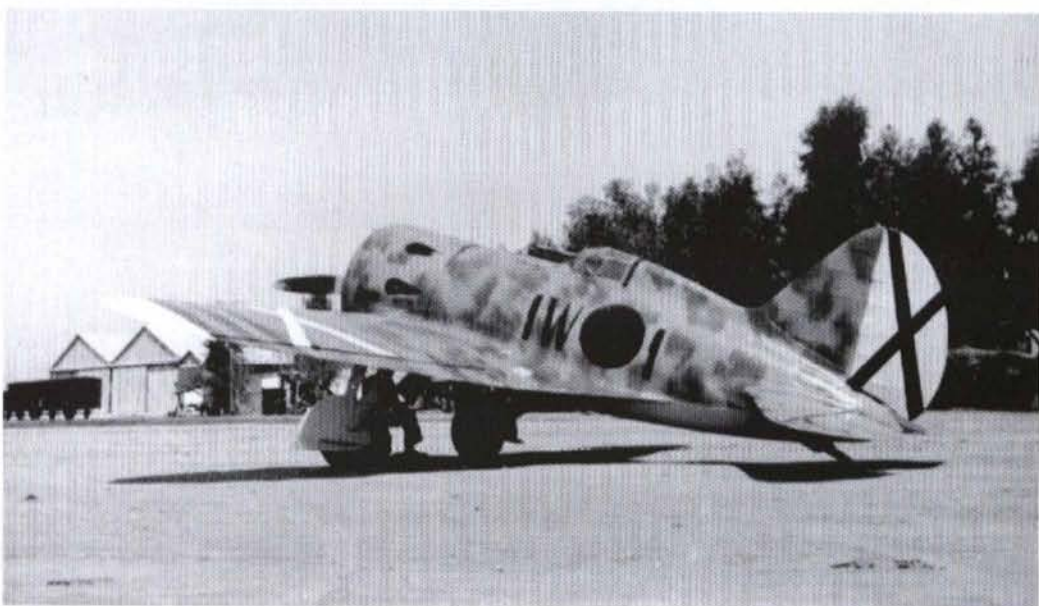
124 Left: Probably the most dangerous enemy to be met in the air by the Legion was the Polikarpov I-16. This Type 5 may be the very first example to be captured by the Nationalists, shown after rebuilding and in service with Grupo 1-W, but it shows all the main features of the airframe. Location is probably Cuatro Vientos 1939
