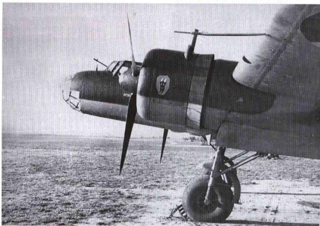
45 Right: Already found in a cruder form on a Heinkel 70, the devil's head emblem of A/88 was painted on the exterior of both engines. The inscription 'Intava' that is visible below the propeller hub relates to the type of oil needed for the BMW 132N radial engines. Note the MG 15 machine gun protruding through the windscreen, probably installed as a result of earlier experience in Spain
