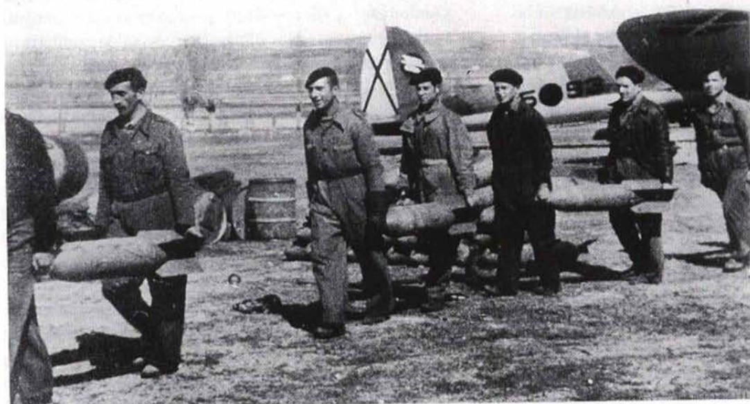
220: Spanish ground crews manhandling German SC 50 bombs. Each He 111 could carry twenty of these, plus a bigger bomb weighing 250kg—and four packs of incendiaries. The work of loading a single machine can be imagined. Behind them is a I.K/88 aircraft, 25-93, which flaunts the unit emblem of a bomb-carrying eagle on the fin. This became the official emblem of I Gruppe of KG 53 in World War II
