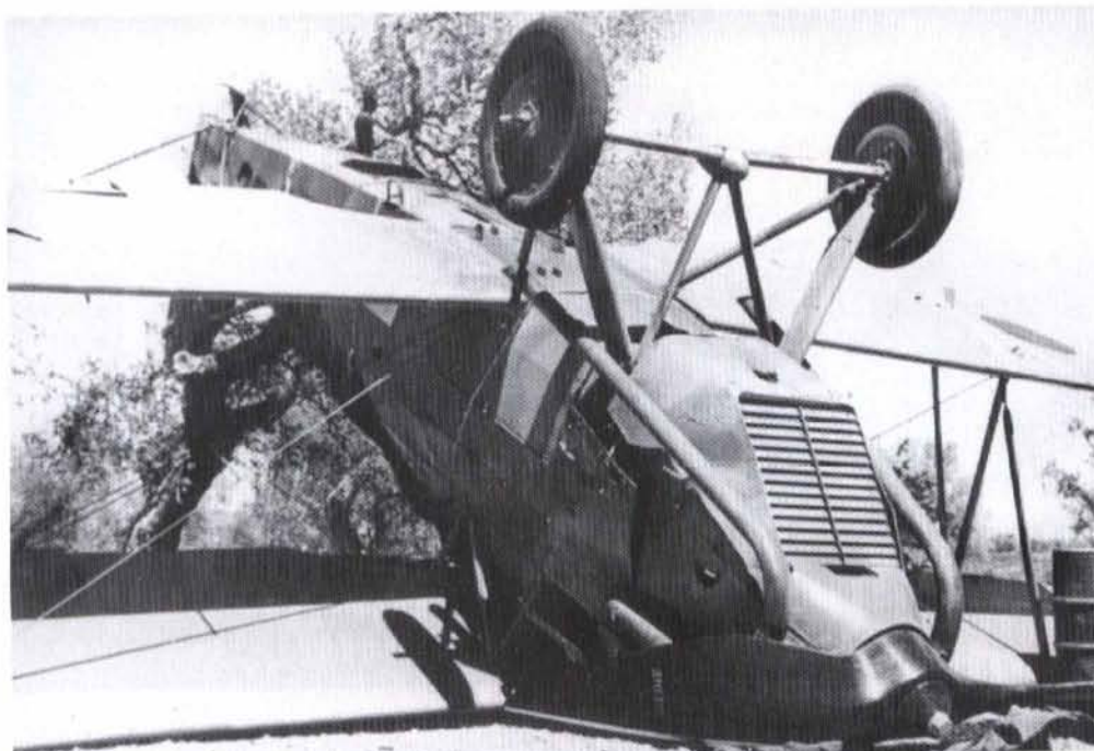
57: Another view of He 45C 15-38 at La Cenia in the morning of 30 August after it had been wrecked in a storm the previous night. The unusual angle allows several underside details to be seen, including the observer's camera hatch and footstep, the radiator louvers in the engine cowling and the Heinkel trademark on the propeller.
