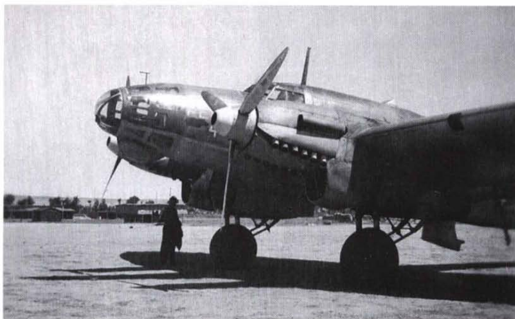
288: A final look at He 111B-1 'Pedro', 25-4, showing the cavernous radiators and 'organ pipe' exhausts of this model. The spinners appear to be white
